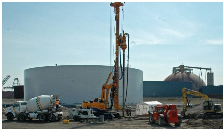
FIGURE 7 Installation of the CMCs in Quebec City.
