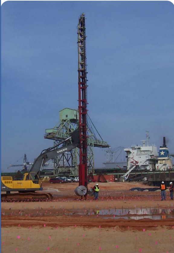
Installing Wick Drains near the port terminal bulkhead.
