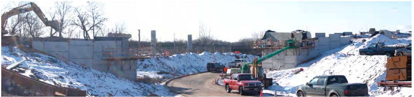
FIGURE 10 view of the MSE Wall under construction
