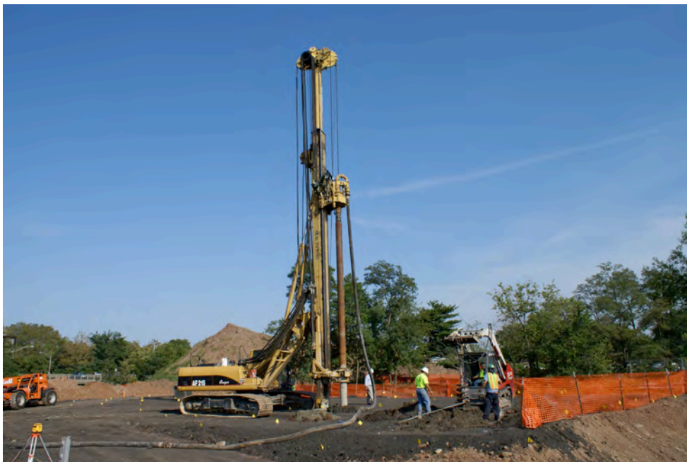
Figure 4 – CMC installation under the MSE Wall
