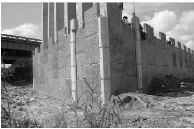
Figures 7 and 8. View of CMC rig and MSE Wall during construction
