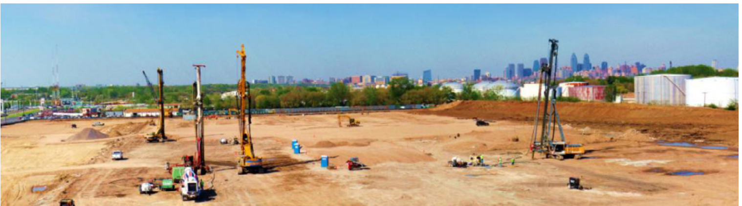
Fig 1: Installation of CMC rigid inclusions
