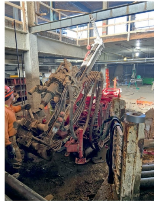
Micropile installation within 4-story building
