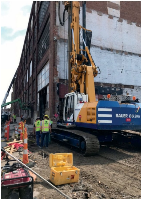
CMC installation near 4-story building façade
