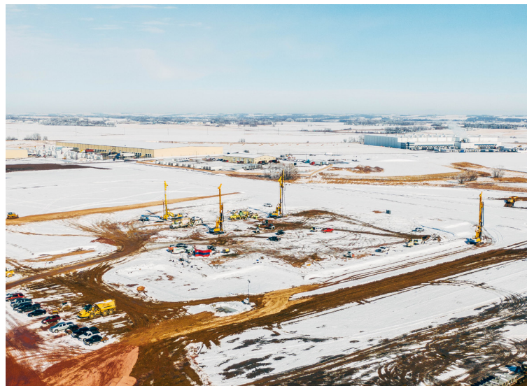
Four drills installing Controlled Modulus Column (CMC)™ Rigid Inclusions to improve ground for a very large distribution center in South Dakota.
