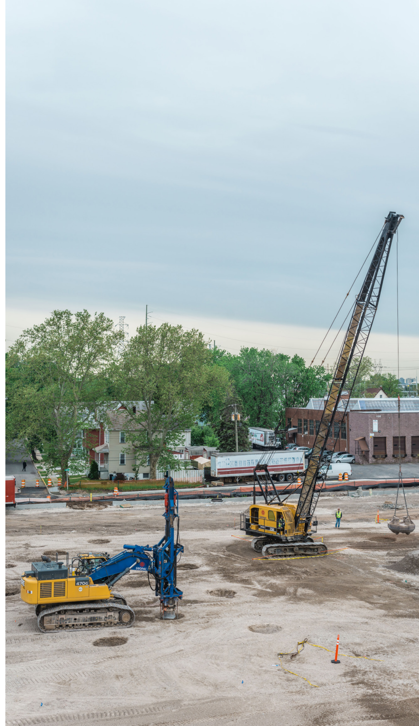
Rapid Impact Compaction (left) and Dynamic Compaction (right) are used to densify fill material to accommodate building construction at a site in New Jersey.
