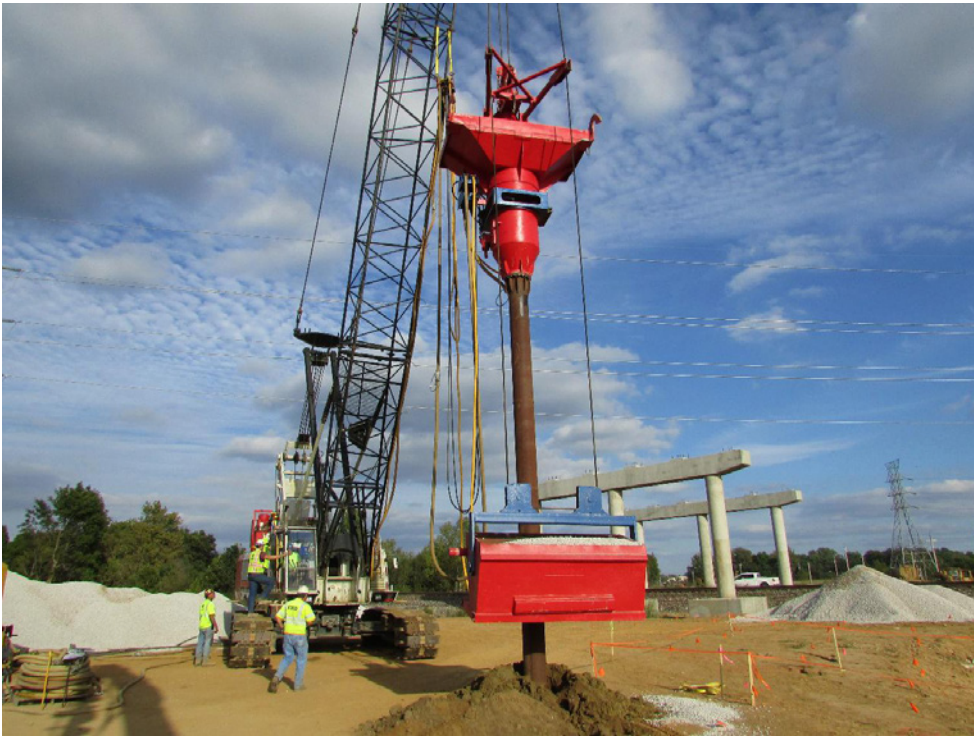
Fig 3 Installation of SCs (dry bottom feed method) and of CMC rigid Inclusions (displacement auger)
