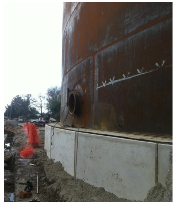
Fig 2: Tank Founded on an MSE/CMC Rigid Inclusion Foundation System
