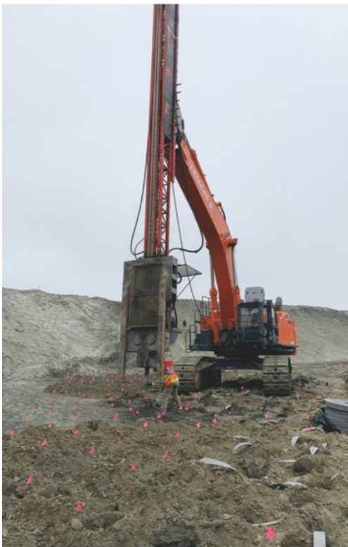
Installation with reattempted wicks in the foreground
