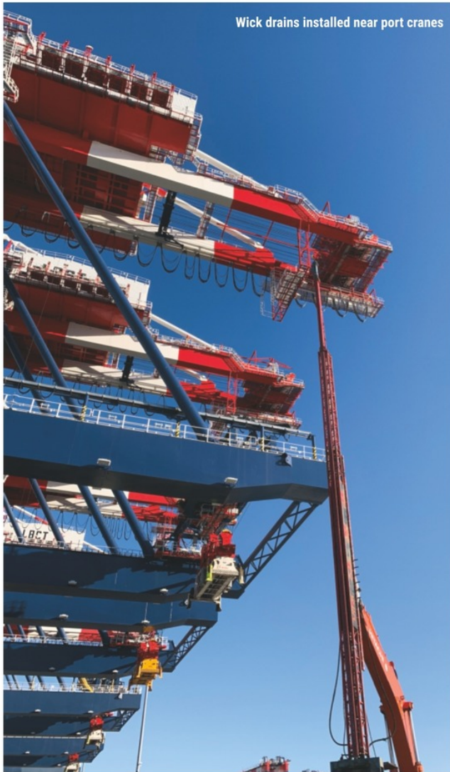
Early wick drain installation
