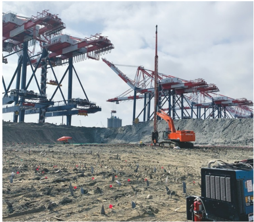
Finishing wick installation in pre-augered holes
