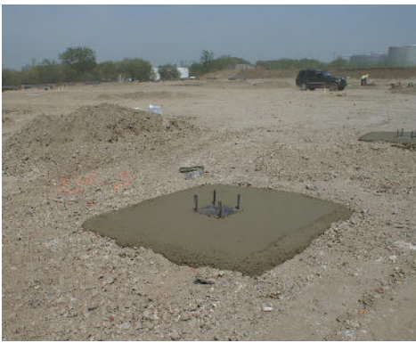
Fig 2: Example of Spread Footing Supported by CMC Rigid Inclusions
