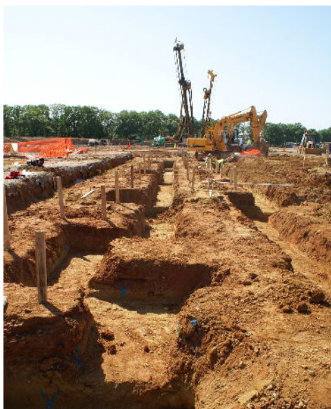
Fig 3: Excavation of Wall Spread Footings After Installation of CMC Rigid Inclusions
